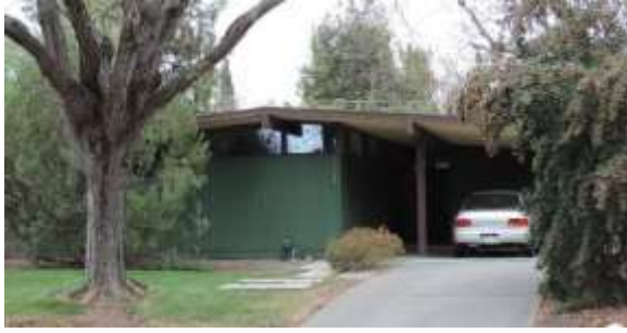
Photograph 25: Post-and-Beam "Classic" at 1128 Princeton Place, 1963
