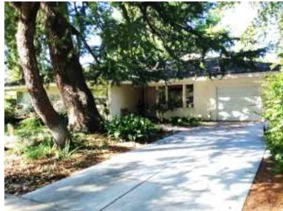
Photograph 11: Contemporary house designed to incorporate passive solar features at 631 Oak Street, 1948. Extreme alterations have obscured the original design.
