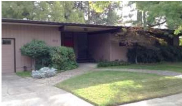
Photograph 32: Custom Ranch house with Post-and-Beam details at 921 West Eighth Street, 1960.
