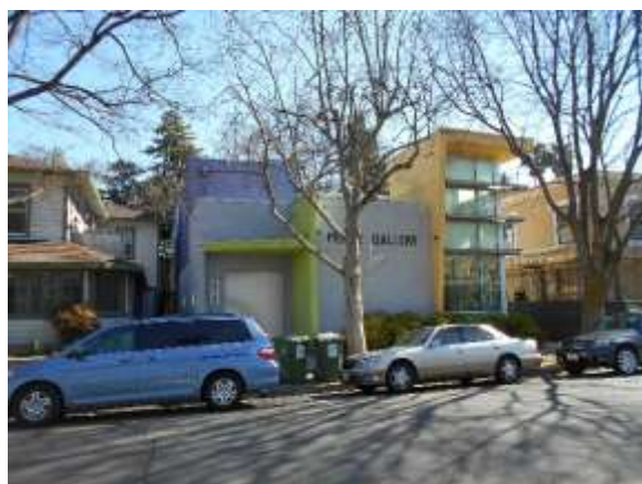
Photograph 2: Contemporary office building at 212 D Street, 1950s. Extreme alterations have obscured original design.
