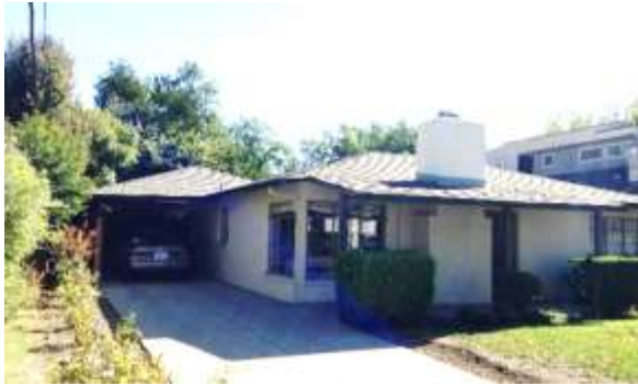
Photograph 8: Hipped-roof Contemporary house with compact plan, decorative chimney, and steel casement windows at 1008 D Street, 1950.
