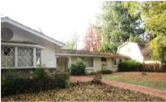
Photograph 31: Custom Ranch at 617 Cleveland Street, 1961.
