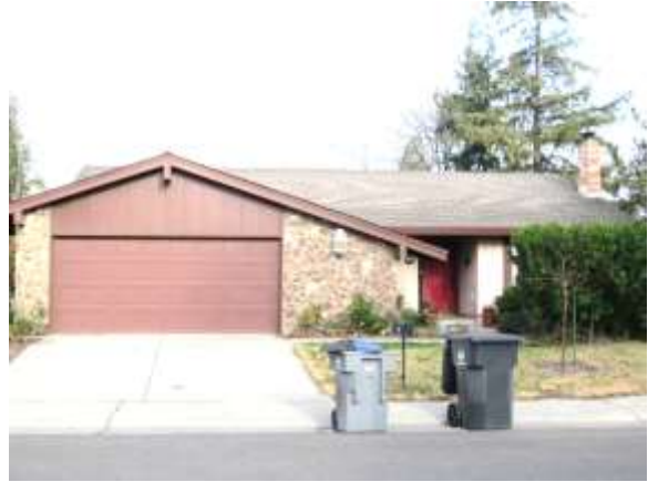
Photograph 42: Custom Ranch house with Post-and-Beam detail at 305 Encina Avenue, 1975.
