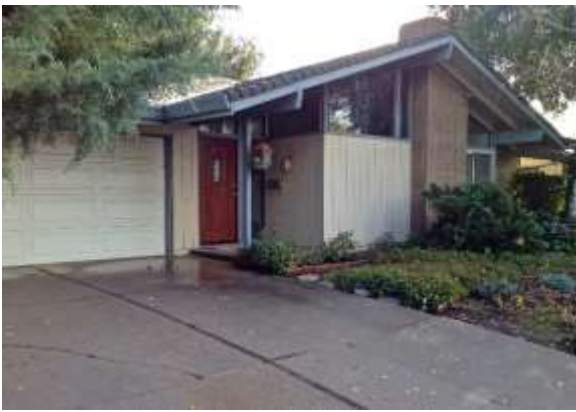
Photograph 27: Post-and-beam transitional house with prominent chimney at 1520 Sycamore Lane, 1971.
