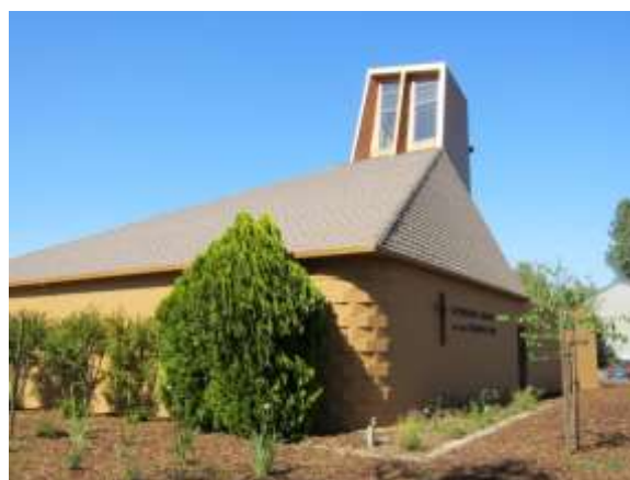
Photograph 20: Lutheran Church of the Incarnation designed by Ostwald and Kelly, 1967.
