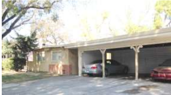
Photograph 15: Three-unit building at 1731 – 1735 Lehigh Drive, 1957.
