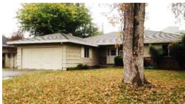
Photograph 23: Hipped roof Tract Ranch house at 825 Acacia Lane, 1966.
