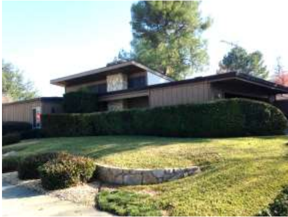
Photograph 39: Custom Contemporary house at 504 Del Oro Avenue, 1972.
