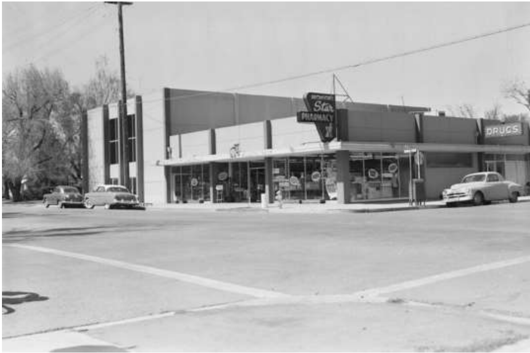
Figure 9: Intersection of Second and D Streets in Downtown Davis, 1957 (Eastman Collection).
