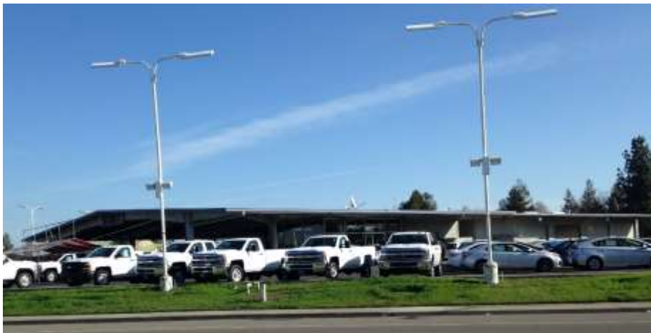
Photograph 38: Post-and-Beam car dealership at 5000 Chiles Road, 1974.
